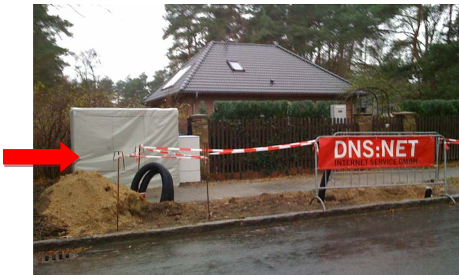
DNS:NET Outdoor-DSLAM am T-Com KVz
